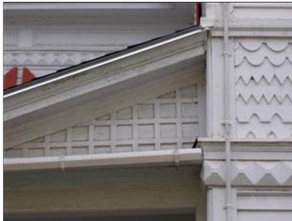
2.3 Picture 3 rear porch settling
