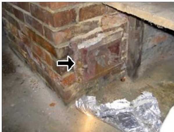
Item 27 - Picture 1 flue clean out door
