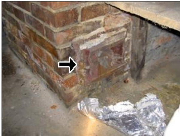
11.5 Picture 1 flue clean out door
